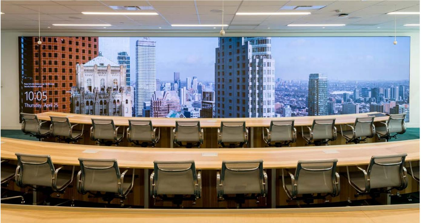
At the center of this focus is a 30-foot-long, 9-foot-high Leyard® DirectLight® X LED Video Wall System in a 20x7 configuration from Leyard and Planar, a Leyard company, that is installed in the auditorium of the Toronto headquarters.
