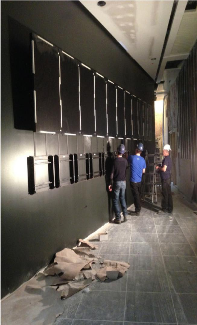
Utilizing Peerless-AV's DS-VW765-LAND mounts, Cablage Expert installed a 4x3 video wall comprised of 55" landscape displays opposite the duty-free area of the international terminal. The 4x3 video wall showcases general information about the airport. Cablage Expert also used Peerless-AV's DS-VW765-POR mounts for an 11x2 video wall, a 2x2 video wall, and a tripod digital signage display.
