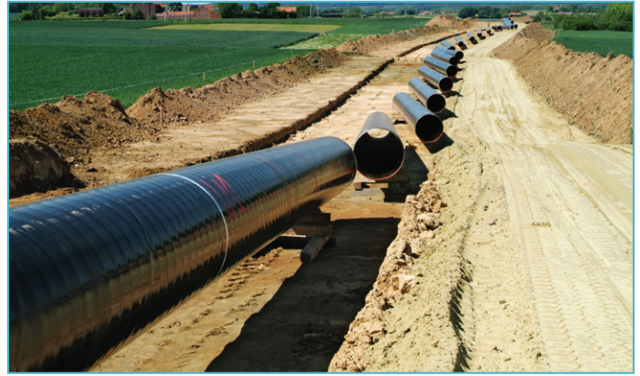
Matrox technology helps Fluxys to oversee thousands of kilometers of high-pressure natural gas pipelines network.
